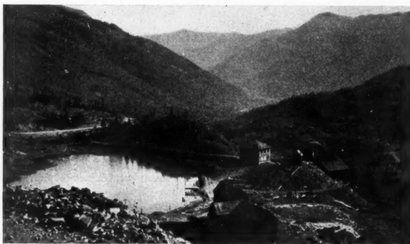
AT THE PORTAL of the Treasury Tunnel in the Red Mountain District of Colorado. The lake is fed by water from the tunnel
